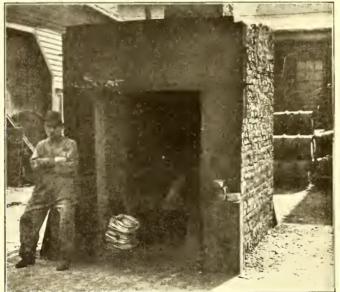
FURNACE FOR BURNING INSULATION FROM OLD WIRE
